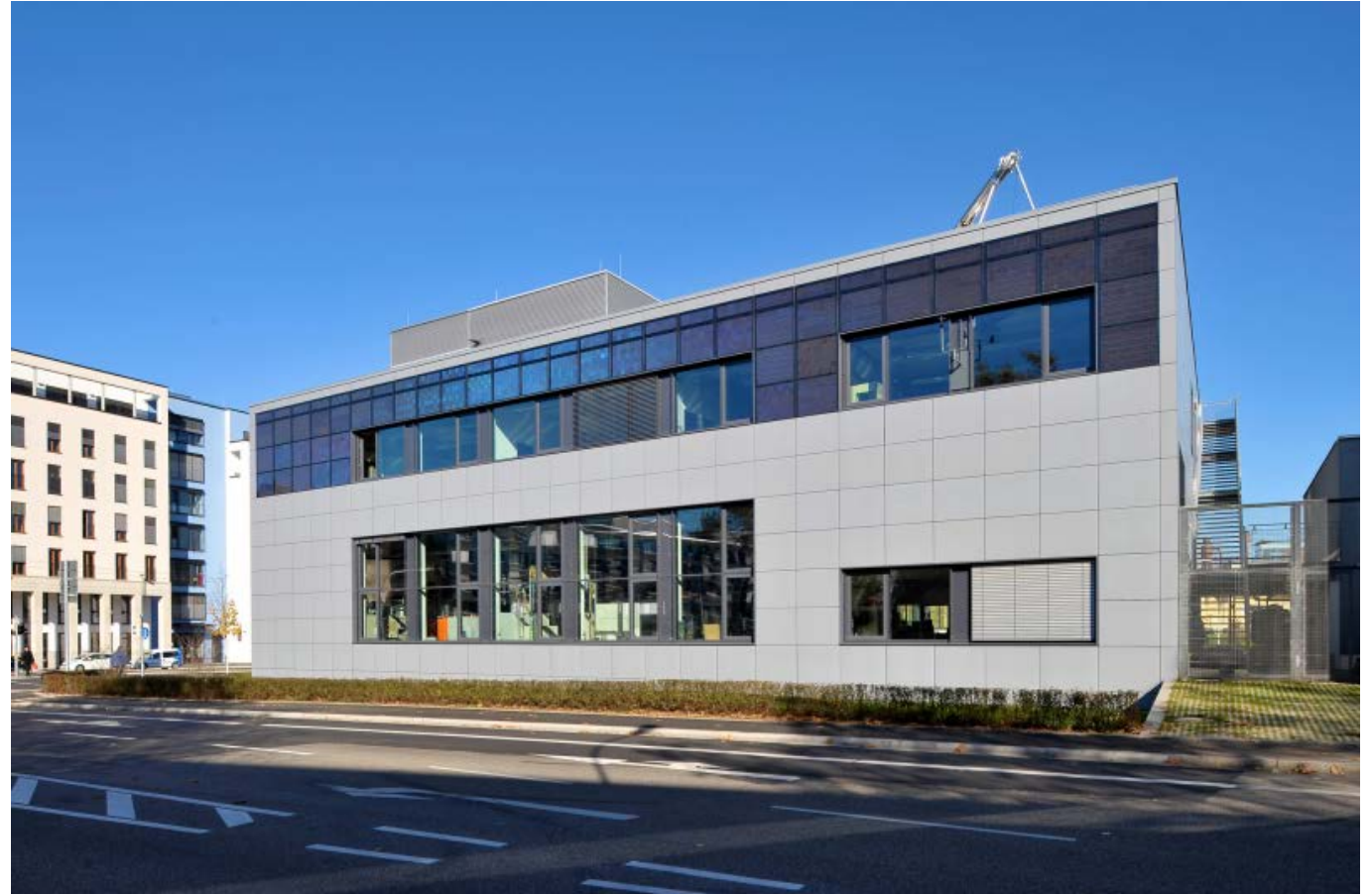
BIPV: Laboratory façade (ISE)
